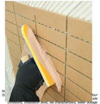
in mixing, cleaning steps and curing conditions. Trial is recommended to verify the application and final colour of the product prior to applying in large scale, especially for stainable tiles and stones.
